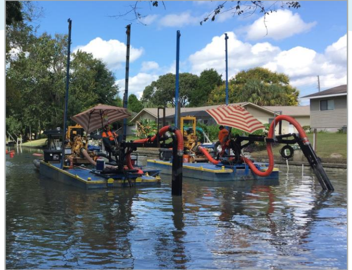
Manatee-friendly modified “suction barges” with mechanical and hand-held hoses were used to remove Lyngbya but not the natural sediment.
